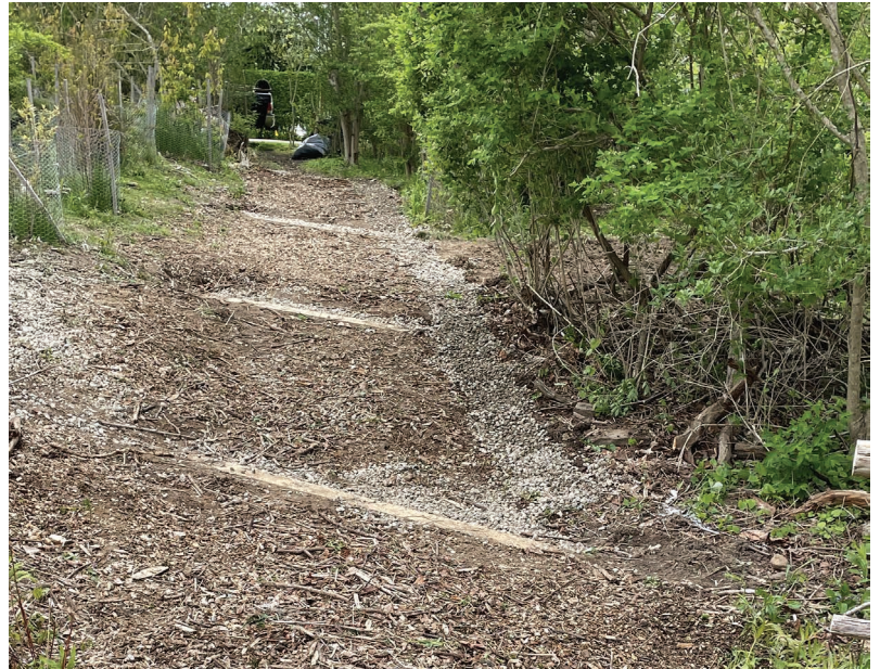
Completed trenches and water bars
