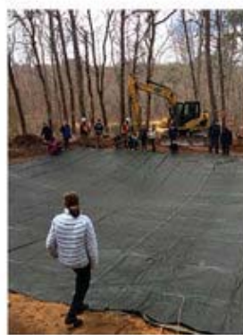
Workers install a protective barrier.
