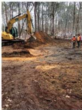
The pools were built in April 2015.
